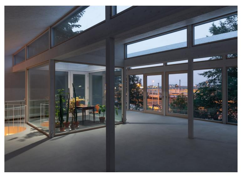
Casa CCFF is an eco-friendly urban house overlooking Geneva's industrial train station. Using low-cost materials and prefabrication, it reduces the construction costs to a minimum. Developed with engineer Marc Walgenwitz, the house is built almost entirely in wood, pushing the structural capacities of this natural material to the limit and reducing the use of concrete to a bare minimum.
