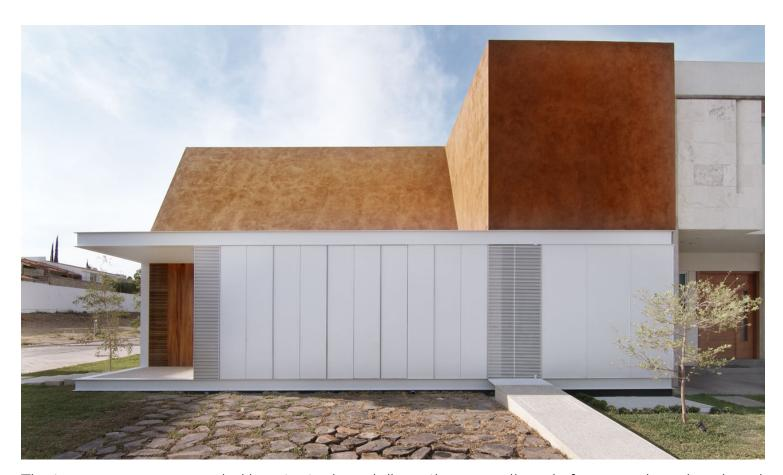
The two cores are surrounded by a tectonic and discontinuous wall made from panels and enclosed by two beams, which support the double-height areas. This white exterior emerges as a base, generating courtyards for day areas and private areas, and highlights the contradiction between the lightness of the tectonic base and the heaviness of the stereotomic volumes, which rise to the height of neighboring buildings, topping off the structure.
