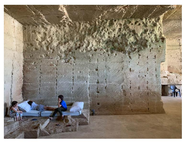
Behind the scan is the architect's eye, directing, interpreting, creating the space again, completing it with operations that are familiar to the stone mass: new cuts to build using air and light. Three skylights are carved into the darkest corners to naturally illuminate and ventilate the space. Stone surfaces are thoroughly cleaned to remove the accumulated mold and dirt. Translucent curtains are introduced to delimit areas of intimacy.
