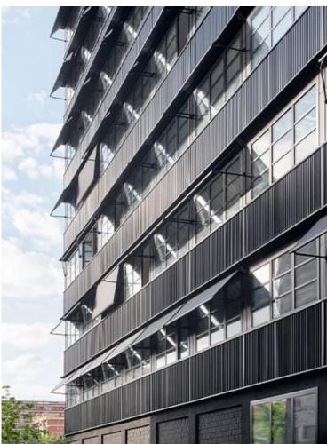
Construction was divided between on-site foundations and ground floor works, and off-site prefabrication of 104 fully equipped 3D modules. This hybrid method significantly reduced construction time—modules were installed in just 15 days, and the total project was completed in 13 months. Factory assembly ensured strict quality control, minimal material waste, and optimized logistics.
