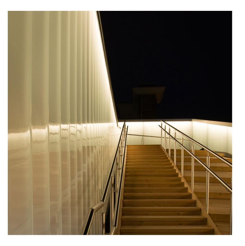
The glass walls are constructed using U-Glass profiles, which are self-supporting and require no metal profiles. The assembly of the glass walls leaves a small gap between each profile, generating a permeable element between the street and the bicycle parking. This provides a sense of safety to the users.
