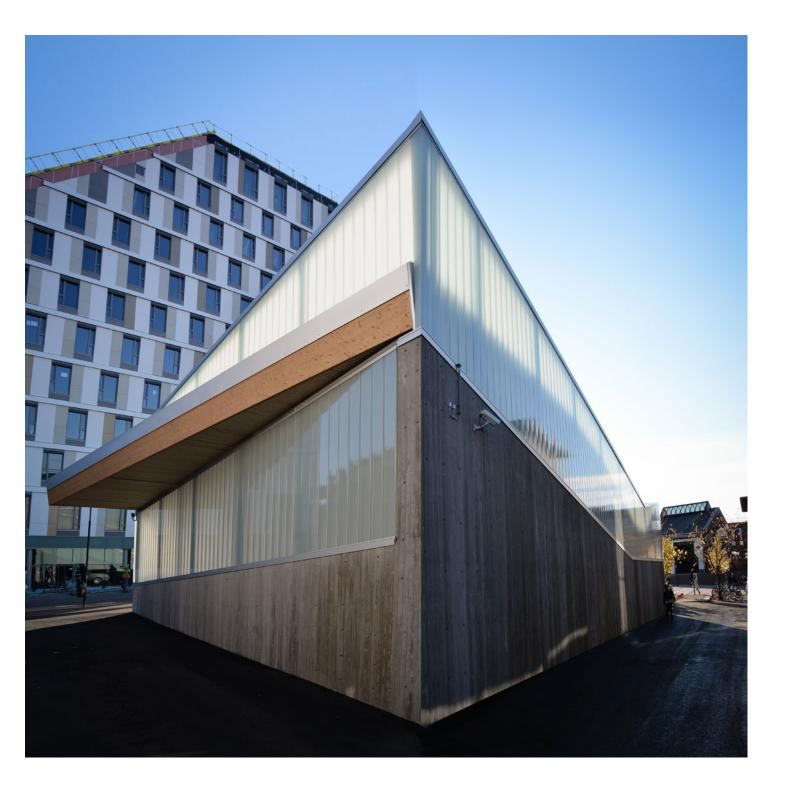
Wood is used for the roof surface, for the furnishings and as a structural material in the curved timber beams. Wood is chosen for its environmental qualities, in addition to the gentle interaction it provides with the public.
