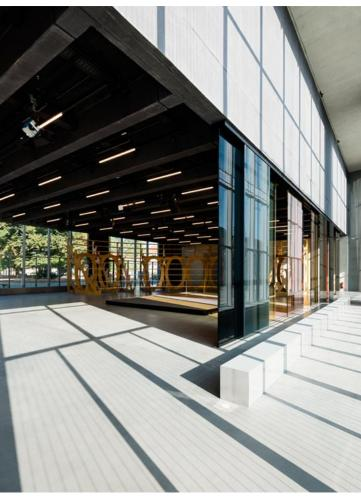
For the load-bearing structure, addenda architects took their cue from bridge building and pushed things to the limit. The cube thus rests only on two stairwell shafts, 50 meters apart, and there are no intervening supporting pillars. The two ends project about 18 meters over the stairwells. Beneath them, on the north side are office spaces and the delivery bay for art and, on the south side, event venues and education spaces.
