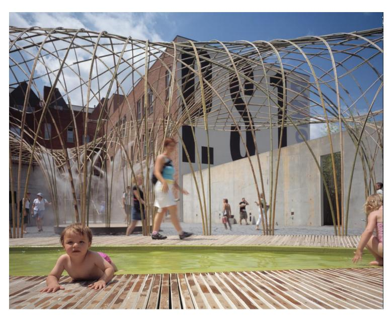
Since *Canopy* was designed as a three-dimensional structural network, the arcs were subjected to more stress during erection than in the final stage. The architects devised a phasing sequence that optimized the structural capabilities of bamboo and minimized breakages. Starting with small areas of the canopy, the team erected structural spanning arcs first and non-supporting arcs second, repeating the sequence until the overall shape had developed. Each arc was assembled on the
