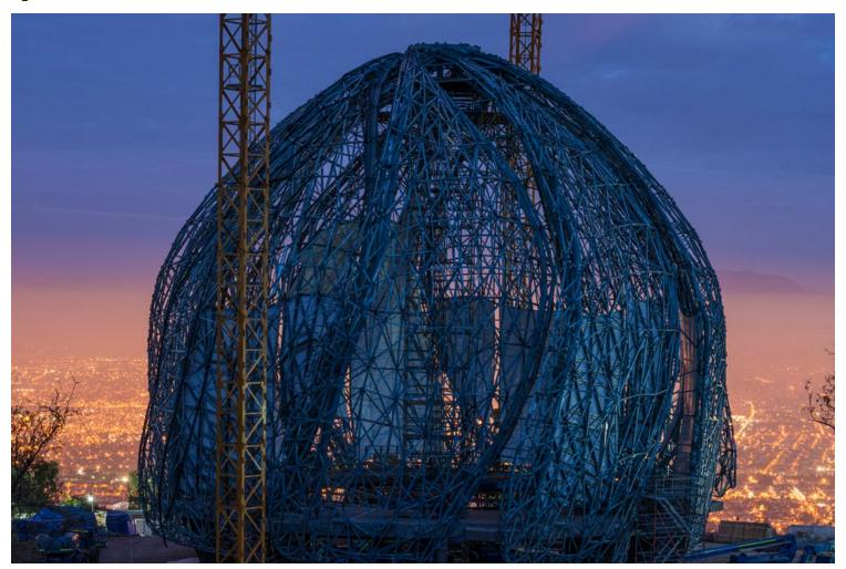
The super-structure of the wings is comprised of hundreds of unique, individually engineered slim-profile steel members and nodal connections. Each of the wings rests on concrete rings and columns set on elastomeric seismic isolators, so that in the event of an earthquake, the concrete pads slide horizontally to absorb the shock.
