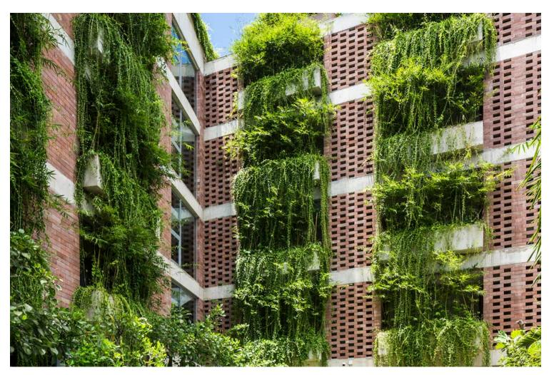
The building façade is clad with locally sourced sandstone pieces used in combination with an exposed concrete slab and a series of planters along the corridors. The planters are arranged along the entire façade of the hotel, which not only provides solar shading but also allows cooler air to ventilate the spaces.
