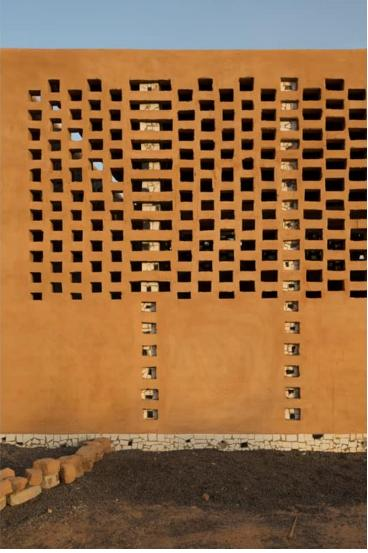
One of the premises of the project is to work with local materials and techniques, which is why the initial excavation becomes the work quarry. By transforming the earth of the site, we managed to reduce the transport of material to a minimum and, with it, the associated ecological footprint.
