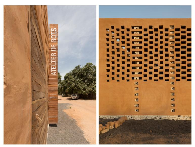
One of the premises of the project is to work with local materials and techniques, which is why the initial excavation becomes the work quarry. By transforming the earth of the site, we managed to reduce the transport of material to a minimum and, with it, the associated ecological footprint.
