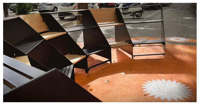
Four movable iron elements make up the arena; they are transportable thanks to handles that attach to the lowest step and wheels placed near the heaviest point of the structure. External guides can be used to install a series of wooden planks that function as a connection between the mobile elements. These wooden elements also allow the third step to be used as a support surface, helping to create different seating configurations and post-debate convivial moments.
