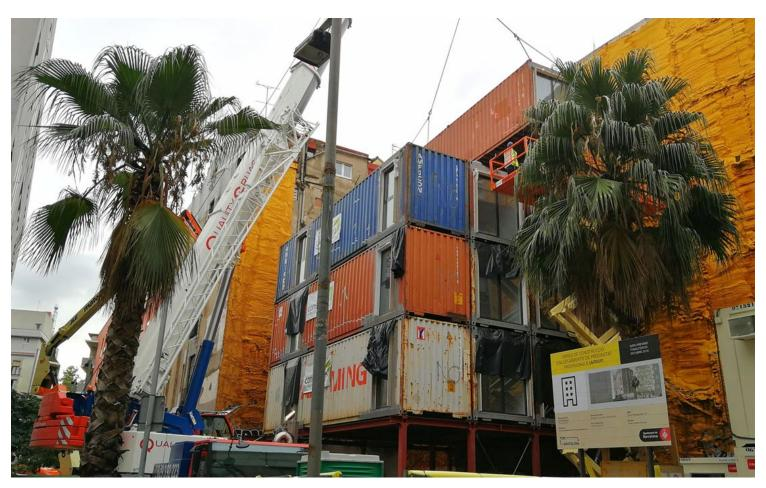
These housing facilities are characterized by the fact that they are modular, transportable and removable, which allows for quick mobilization of empty spaces in the city for different time periods. These buildings can also incorporate some public facilities or spaces for community use.
