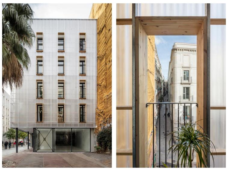
Around this compact volume, a translucent polycarbonate façade is projected that responds to the alignments of the plot. This second skin serves as a separator between the outside environment and the containers, with climatic, spatial and visual features. On the east façade, facing historic buildings, the openings in the polycarbonate skin adapt to the character of the neighborhood, with vertical
