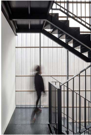
The circulation core is strategically placed next to the party wall, providing a convenient interaction with the neighboring building and guaranteeing access to all units through gateways that are large enough to allow other uses besides transit. The translucency of the polycarbonate skin also
