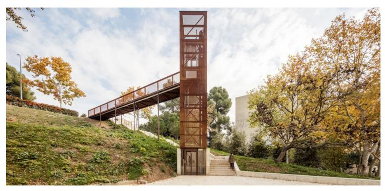
The proposal consists in installing a lift in a strategic point that makes it easier to see and reduces the distances people have to walk. The structure consists of a framework of tubular metal 10-cm profiles and diagonal 5-cm profiles.
