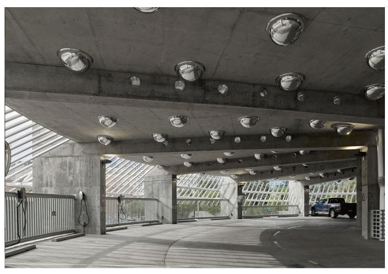
The structure is enveloped in a distinctive guard shroud, raised strategically around the perimeter to provide pedestrian, bicycle, and vehicular access. The members of the shroud hold a fine-grained mesh that acts as a pedestrian guardrail today, while easily and inexpensively accommodating conversion into residential/commercial suite balconies with no additional work required.
