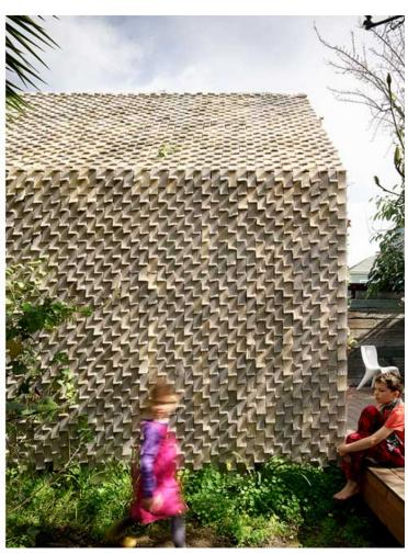
The roof and contiguous facades to the gable are clad in a 3D printed ceramic rain screen of seed stitch tiles—a 3D-printed ceramic cladding system that serves as a rain screen. Designed for easy assembly, the <u>Seed Stitch</u> tiles are made to be hung on a building facade or interior. The surface of each ceramic tile visually emulates a knitting technique called the seed stitch.
