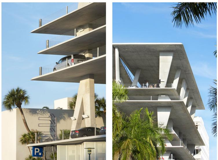
The structure is the architecture. The car park is an organism made up of a family of concrete slabs, deployed as floor plates, columns and ramps. The location and form of these elements result from a series of forces acting upon each other, a complex overlapping of site and building code requirements, combined with program choices and the aspiration to both integrate with Lincoln Road Mall and to formulate its beginning at the corner of Alton Road.
