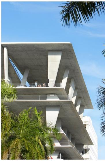
The structure is the architecture. The car park is an organism made up of a family of concrete slabs, deployed as floor plates, columns and ramps. The location and form of these elements result from a series of forces acting upon each other, a complex overlapping of site and building code requirements, combined with program choices and the aspiration to both integrate with Lincoln Road Mall and to formulate its beginning at the corner of Alton Road.
