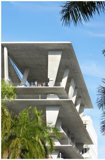
The structure is the architecture. The car park is an organism made up of a family of concrete slabs, deployed as floor plates, columns and ramps. The location and form of these elements result from a series of forces acting upon each other, a complex overlapping of site and building code requirements, combined with program choices and the aspiration to both integrate with Lincoln Road Mall and to formulate its beginning at the corner of Alton Road.
